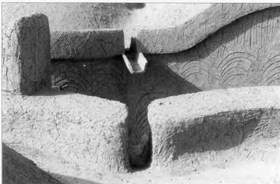
Figure 5 Particular care in shaping roofs to ensure quick but controlled rainwater run-off
