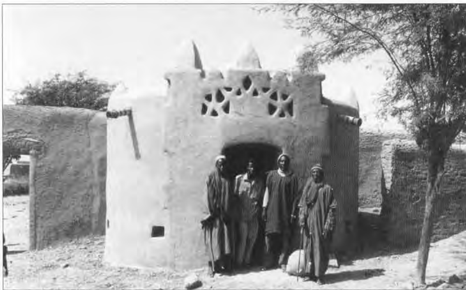
Figure 4 Woodless Construction clients often attach great importance to the final appearance of their building. This round, domed building is finished in the manner locally typical of rectangular, flat-roofed buildings.
