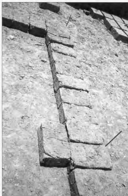
Figure 1 Ordinary mud bricks of local dimensions are used as the unit of measurement in laying out. Increasingly only header courses are used.
