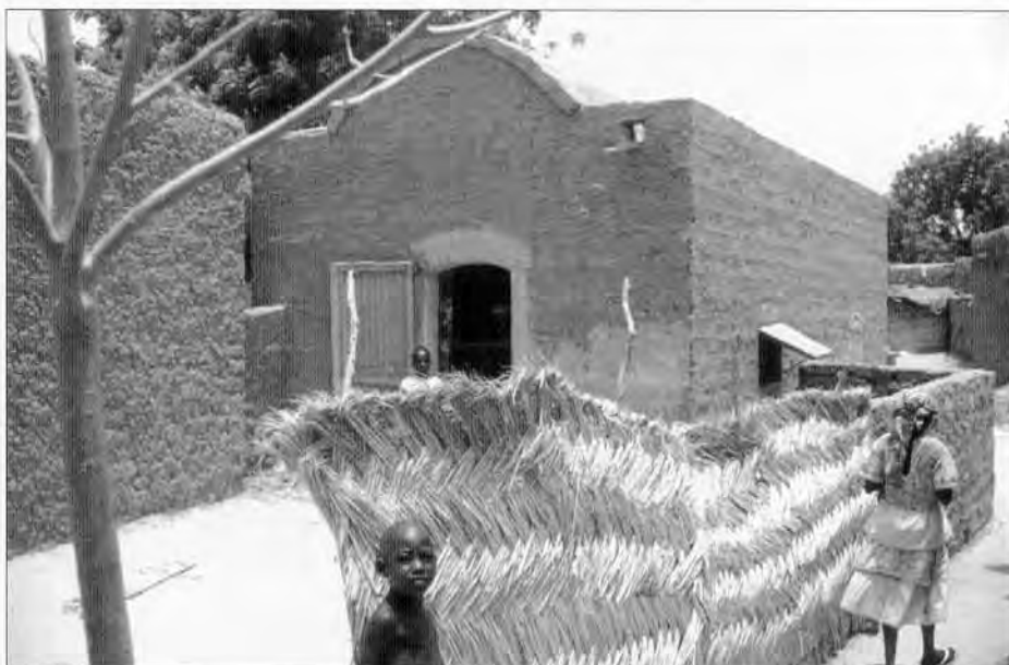
Figure 4 "Spontaneous" construction – a vaulted house built by a trained mason with no external help
