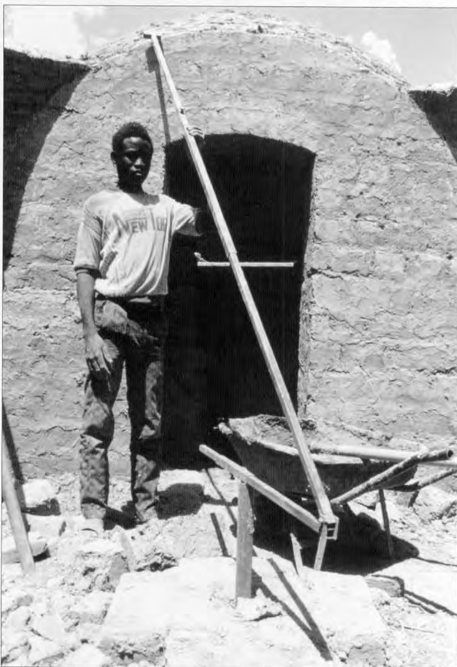
Figure 3 An adjustable radial arm is given to each mason at the end of his basic training, enabling him to build eccentric domes.
