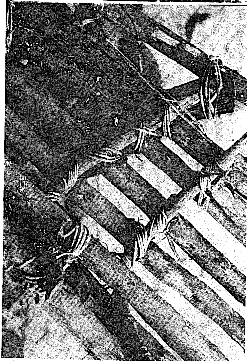
Fig. 79 Lashing using stripped cane, Sau River Bridge.
