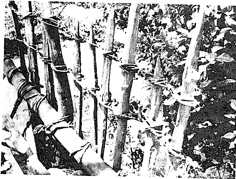
Fig. 63 Abutment scaffolding, Kubib Bridge.
