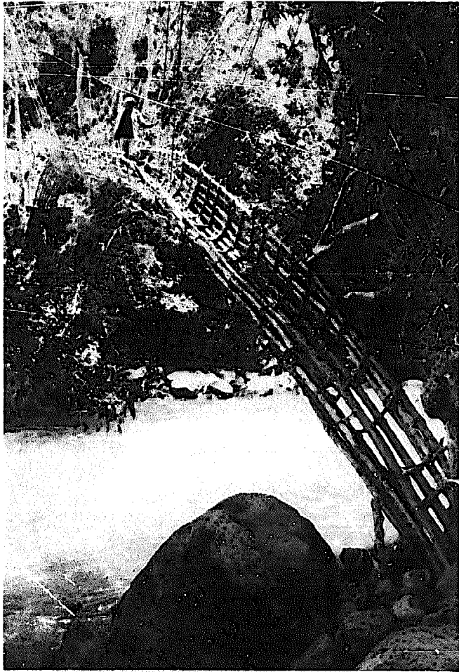
Fig. 76 Sau River Bridge.
