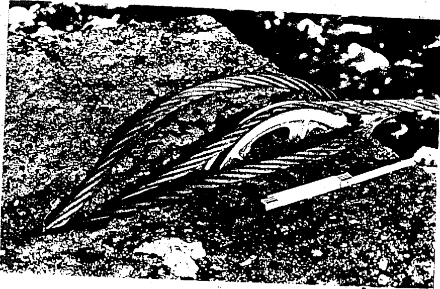
Cable Support Point, Item 1
