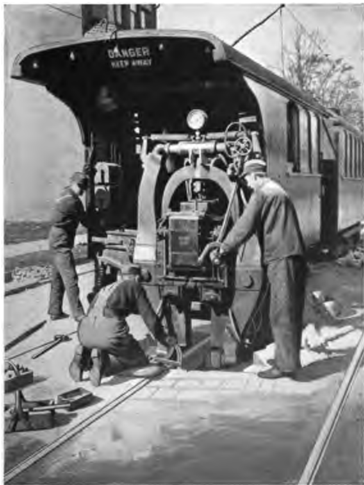
FIG. 262. — Welding track electrically. The equipment consists of an inverted rotary converter to change the direct current of the trolley to an alternating current, a regulator to keep the voltage practically constant, and the welding transformer.
