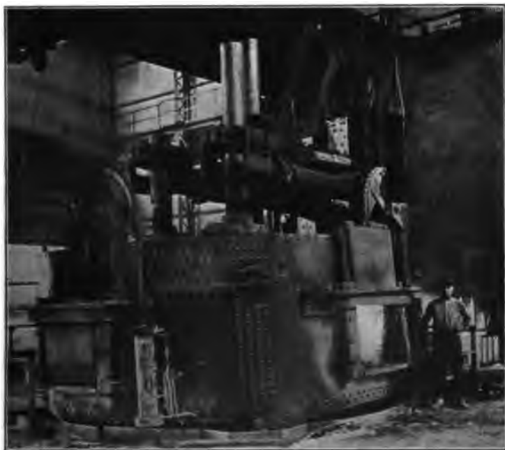
FIG. 344 a. — A 20-ton, 3-phase Heroult electric steel furnace fitted with three 12-inch graphite electrodes.
