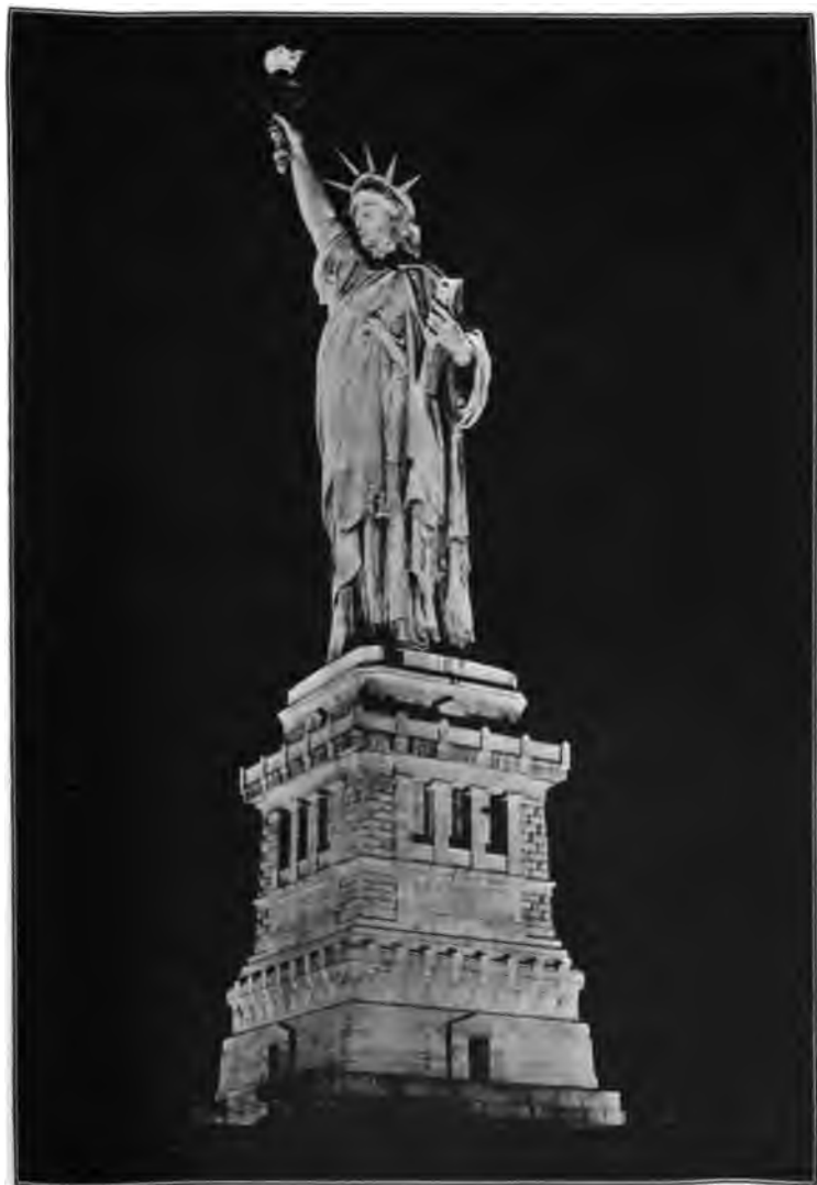
FIG. 334. — Statue of Liberty illuminated at night by means of 15 batteries of flood-lighting projectors using 250-watt tungsten lamps.
