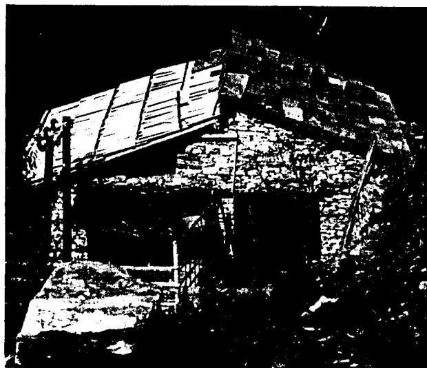
The powerhouse at Barpak
