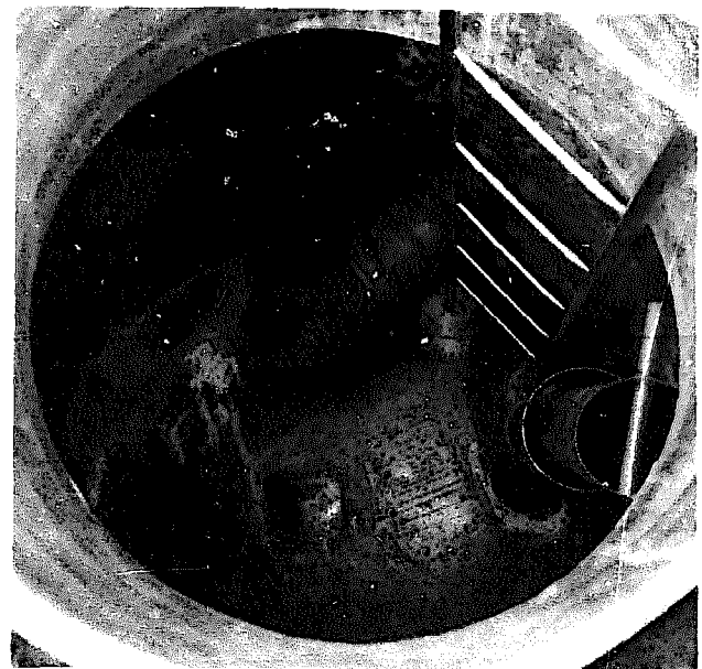
Fig. 18: Surge tank of glass-fibre reinforced plastic (1.5 m dia.) with intake sieve on penstock and overflow via the plugging pipe in the bottom .
