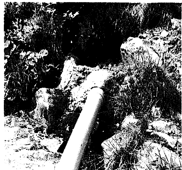
Fig. 8: Spring kerb: Immediately after emerging, the water is collected in a concrete basin and is led into a PVC-pipe (inner diameter 100 mm).
