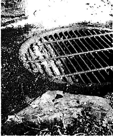
Fig. 13: A simple intake consisting of a trash rack made of concrete reinforcing steel, placed on a concrete pipe (inside dia. 100 cm) which is dug into the bed of the stream.
