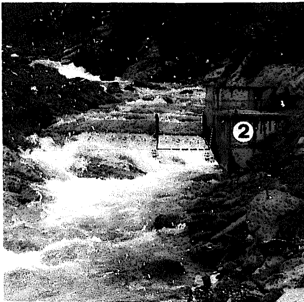
Fig. 15: Water intake and desilting basin in the flat section of the stream. 1 Tirolian type intake (flooded) 2 Desilting chamber
