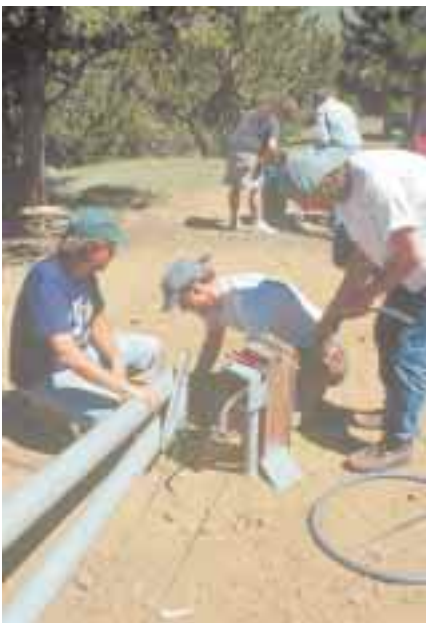
Assembling the tilt-up tower.
