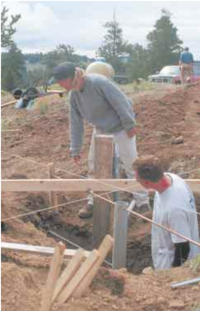
Setting the anchor orientation amidst a cat's cradle of leveling strings.
