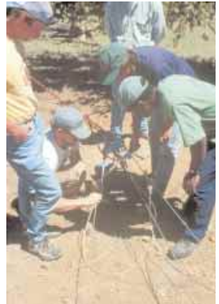
Untangling the maze of tower guy cables.
