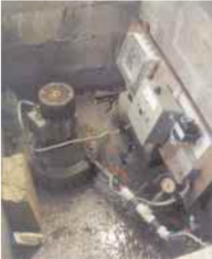
The Bosque del Cabo system utilizes a 1 1/2 HP motor (left) to produce 180 watts from 21 gpm at 190 feet of head. 2,300 feet from the hydro unit, the rest of the system (right) steps down from 415 VAC to 12 VDC.
