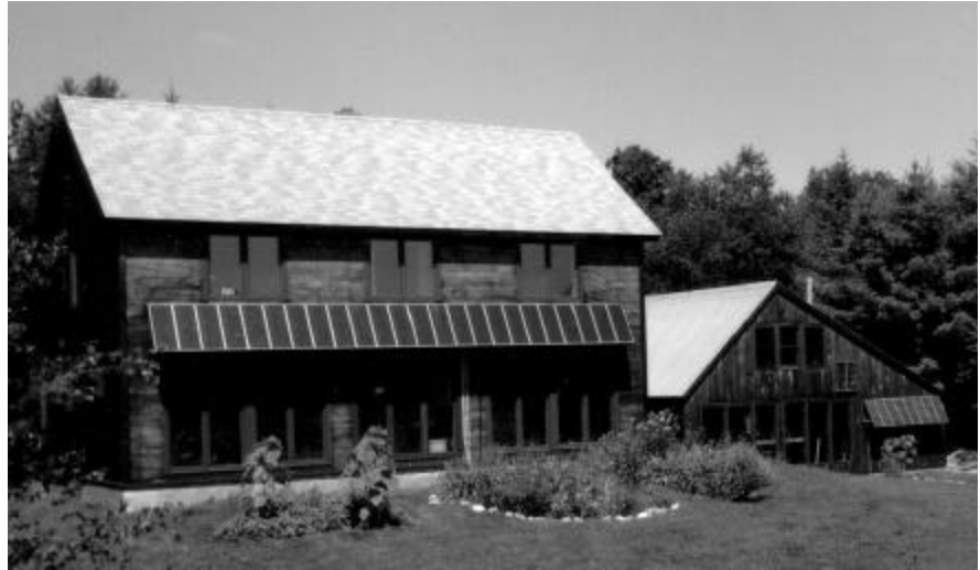
The author's home, with solar electric modules on the house and garage
