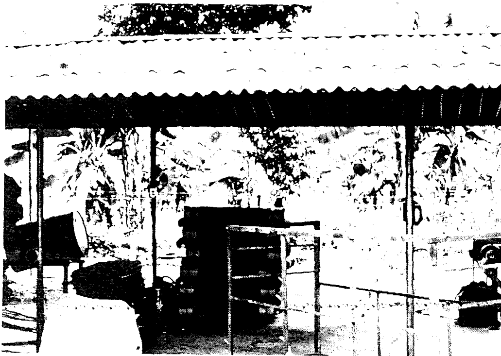
Fig. 12b Finished asphalted sheets in position.
