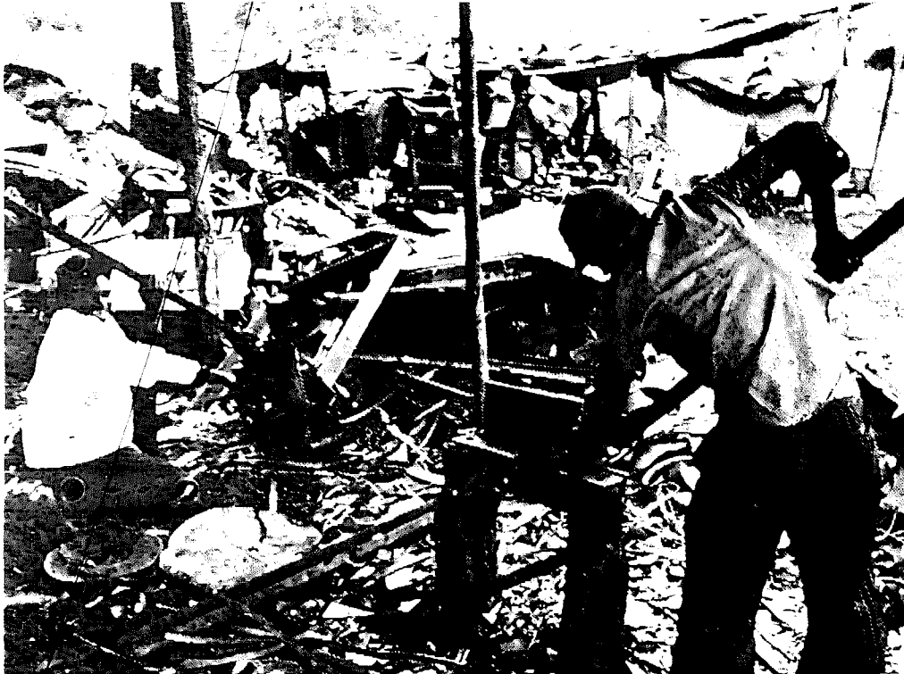
Fig. 20 Hand-made metal forming machines: this workshop included a shear, a punch, a bending machine and a machine for cropping reinforcing bars, all made with a hacksaw, hand drill, etc. Note how the machines have been mounted on wooden trunks, hammered into the ground in the absence of a concrete floor.
