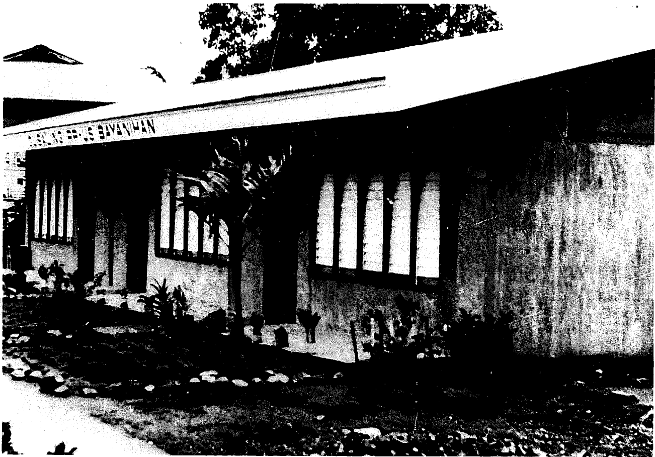
FIGURE 5 BAYANIHAN SCHOOL BUILDING.
