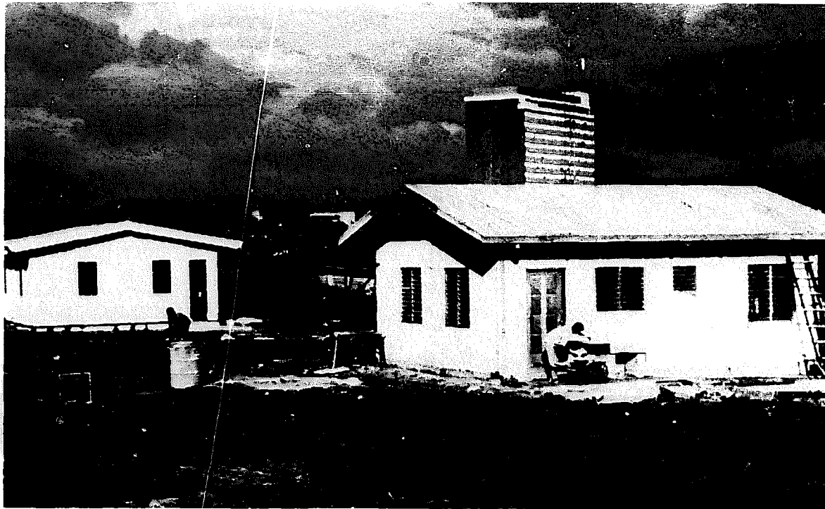
FIGURE 3 TWO TEST HOUSES AT QUEZON CITY SITE.
