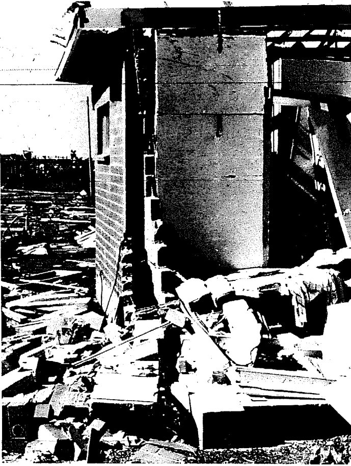
FIGURE 15 BUILDING OF CAVITY WALL CONSTRUCTION IN DARWIN, AUSTRALIA, PARTIALLY DESTROYED BY THE DECEMBER 1974 CYCLONE.
