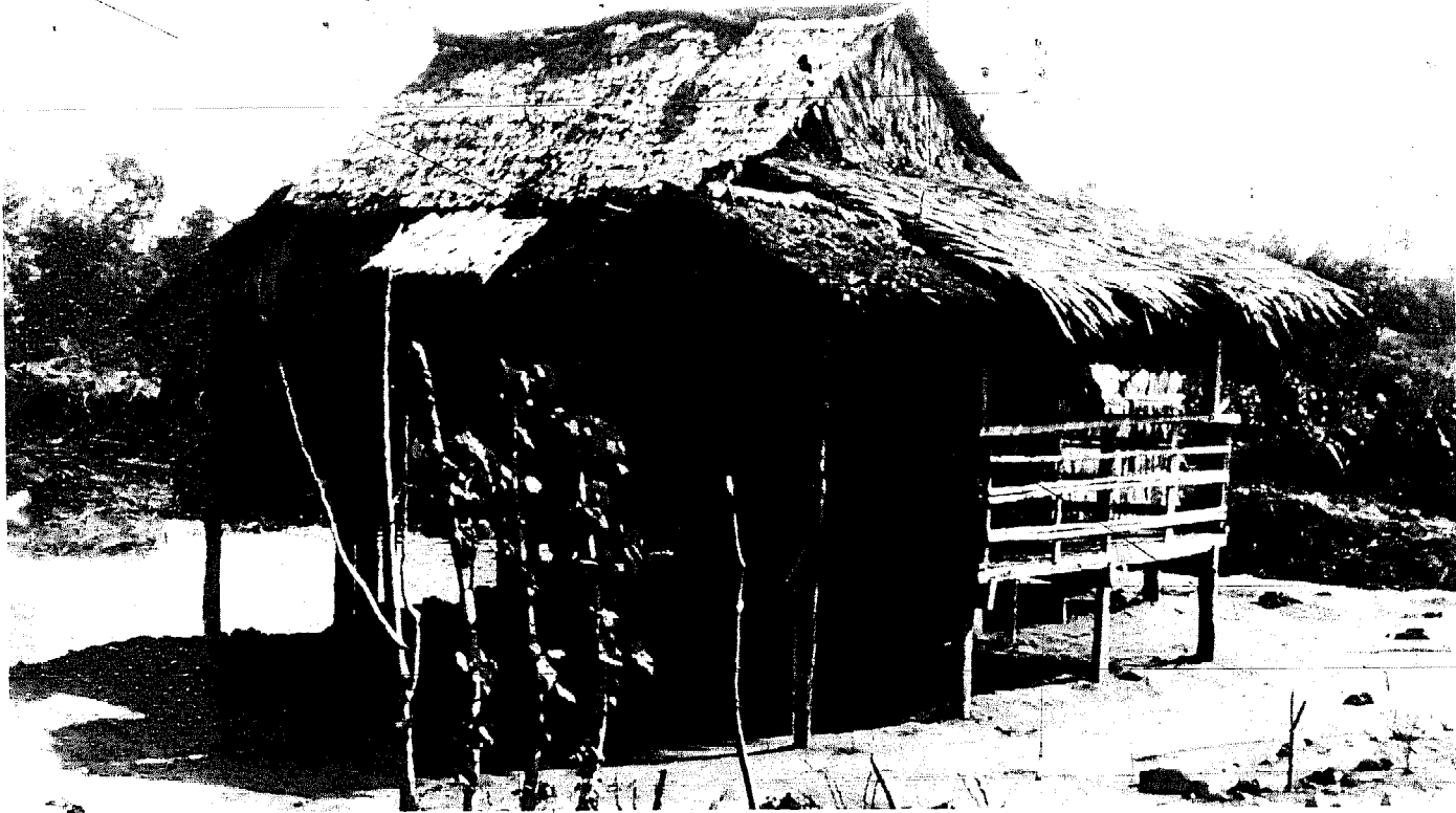
FIGURE 39 POLE-TYPE CONSTRUCTION.
