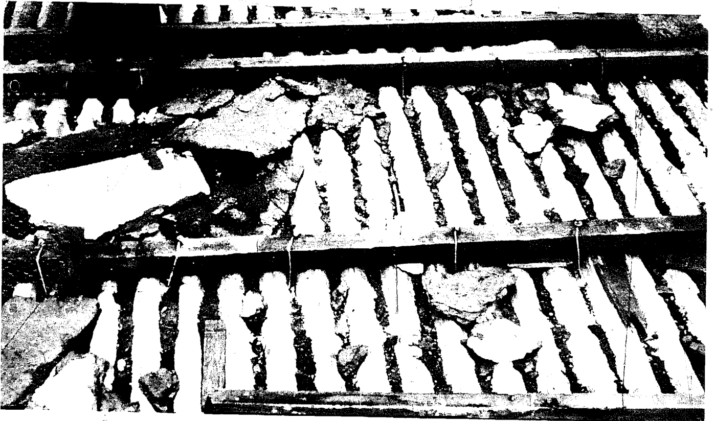
FIGURE 50 ALTHOUGH THE ROOF BLEW OFF OF THE STRUCTURE, THE CORRUGATED ROOFING WAS EFFECTIVELY TIED TO PURLINS BY WIRES COMPLETELY AROUND THE PURLINS.
