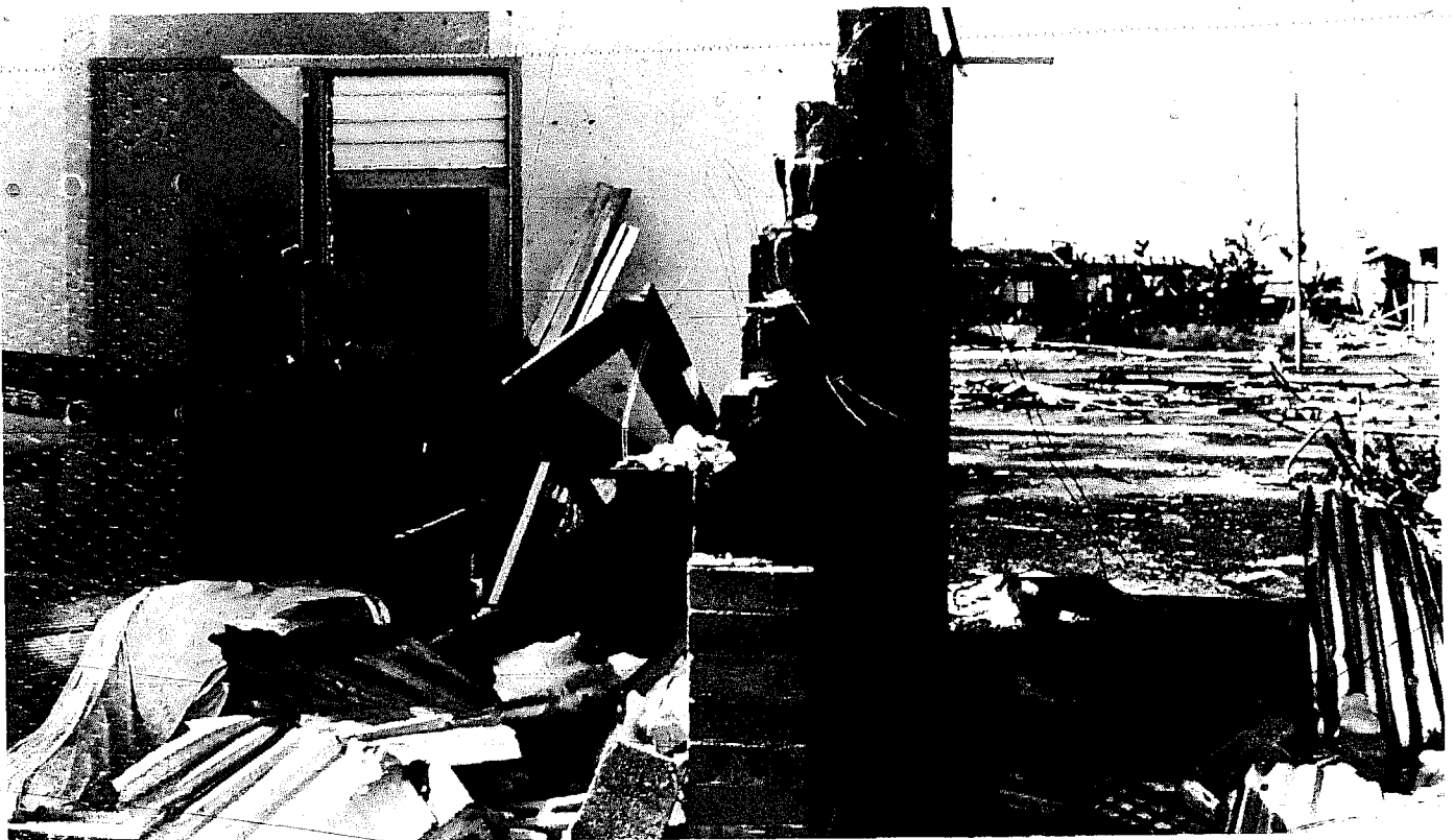
FIGURE 14 RESIDENTIAL BUILDING IN DARWIN, AUSTRALIA, DESTROYED BY THE DECEMBER 1974 CYCLONE.
