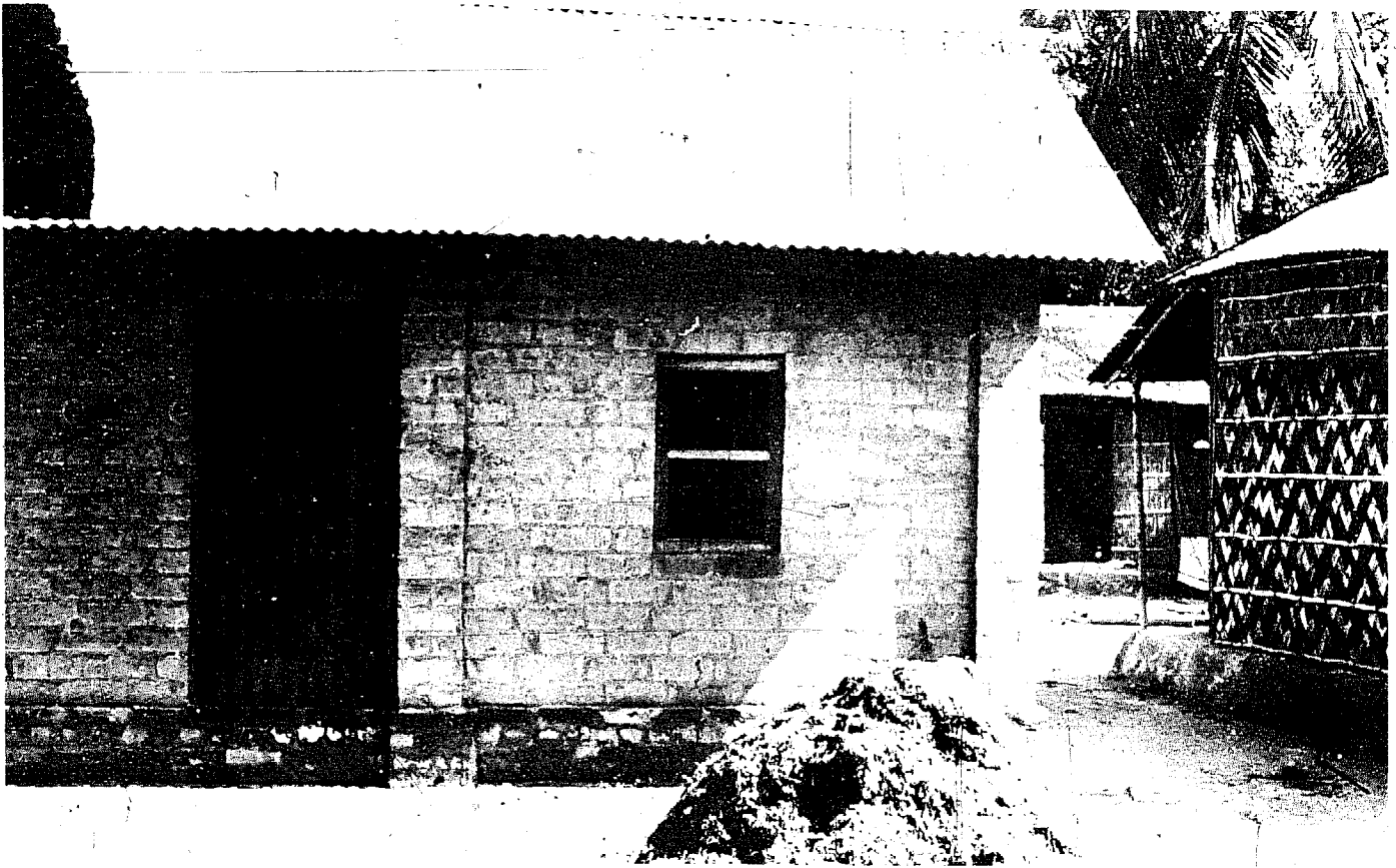
FIGURE 27 CARE SPONSORED HOUSING PROJECT NEAR DACCA, BANGALADESH SHOWING CINVA-RAM WALL CONSTRUCTION WITH CORRUGATED METAL ROOFING.
