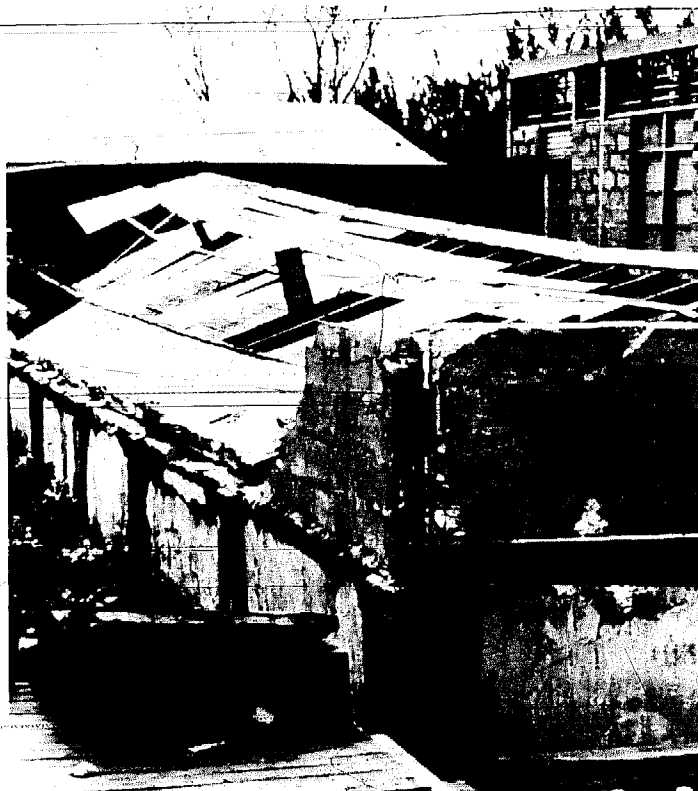
FIGURE 8 COLLAPSE OF ONE-STORY BUILDING CAUSED BY THE NOVEMBER 1974, TYPHOON IN THE PHILIPPINES.
