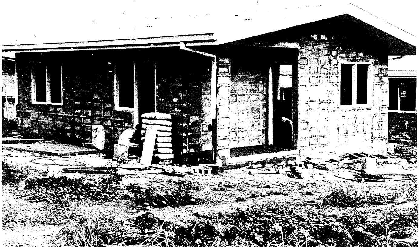
FIGURE 18 SINGLE FAMILY MASONRY HOUSE UNDER CONSTRUCTION IN CENTRAL LUZON, THE PHILIPPINES.
