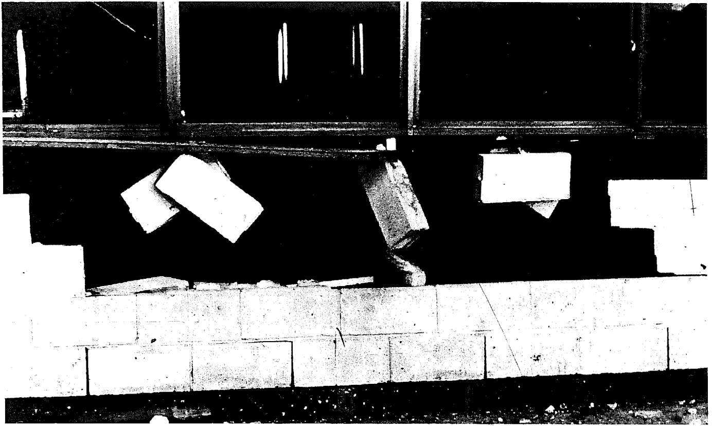
FIGURE 17 FAILURE OF CONCRETE BLOCK MASONRY WALL IN BUILDING SUBJECTED TO THE DECEMBER 1974 CYCLONE IN DARWIN, AUSTRALIA.
