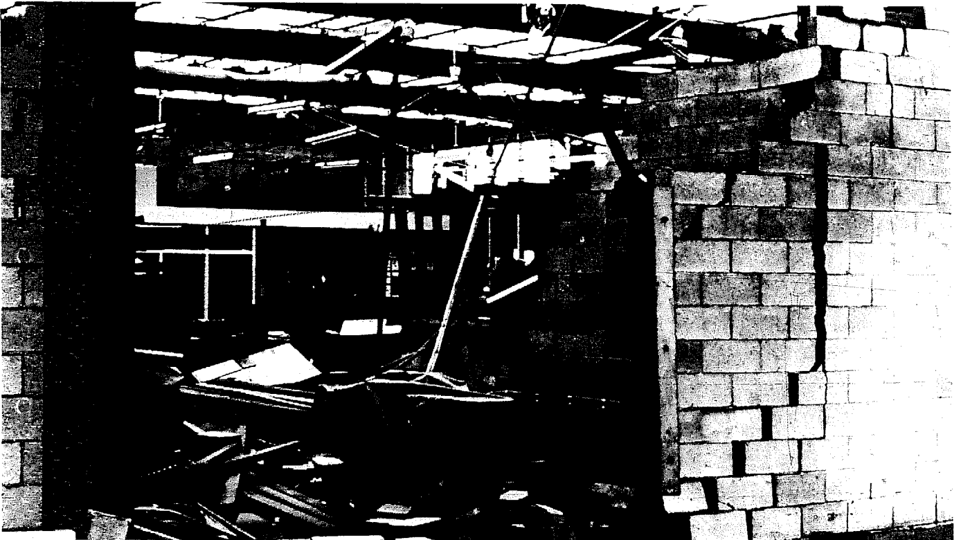
FIGURE 16 BUILDING IN DARWIN, AUSTRALIA SHOWING PARTIAL COLLAPSE OF ROOF AND MASONRY INFILL WALLS CAUSED BY THE DECEMBER 1974 CYCLONE.
