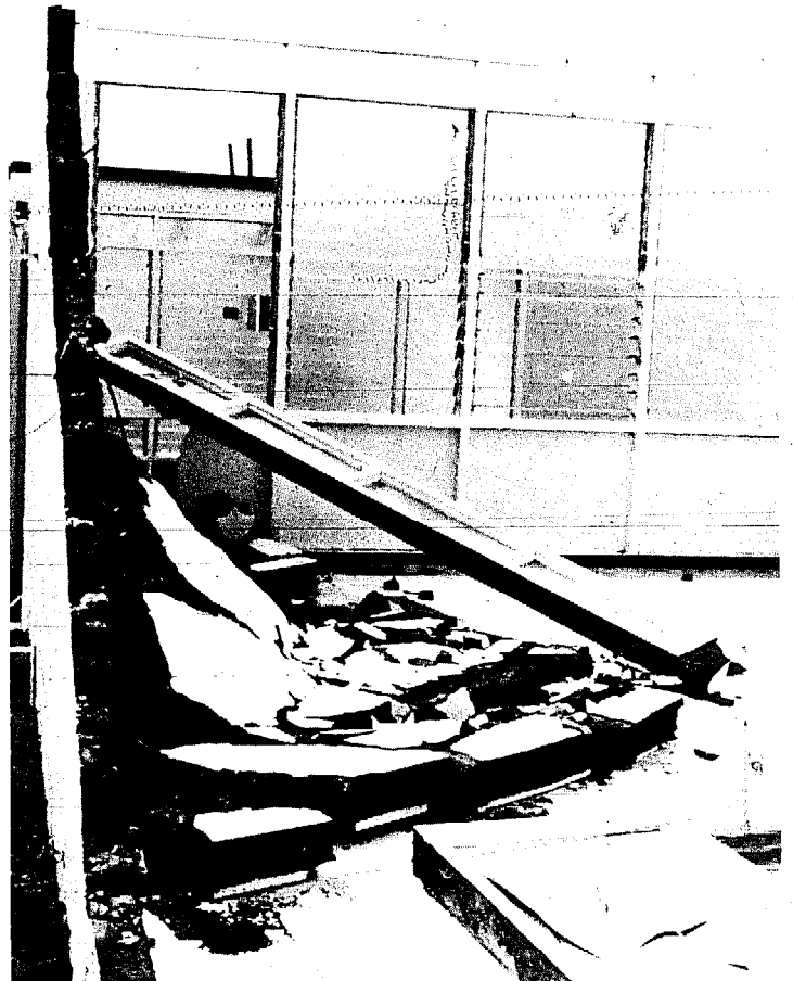
FIGURE 12 SINGLE FAMILY HOUSE SHOWING COLLAPSE OF ROOF AND EXTERIOR WALL DURING THE PHILLIPINES TYPHOON IN NOVEMBER 1970.
