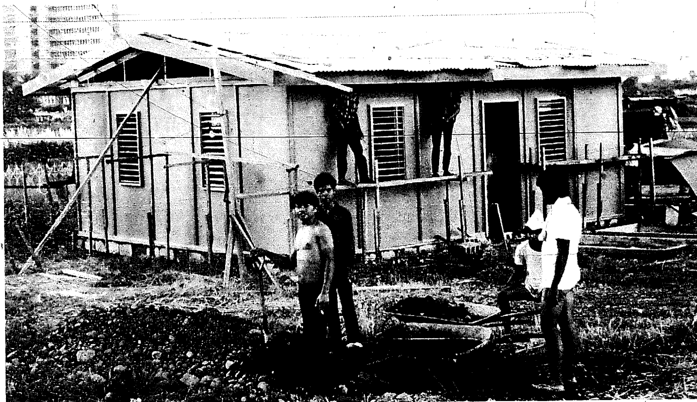
FIGURE 40 WOOD-FRAME WALL AND ROOF.
