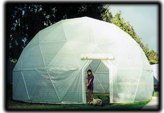
24 ft. dome with opaque greenhouse vinyl
