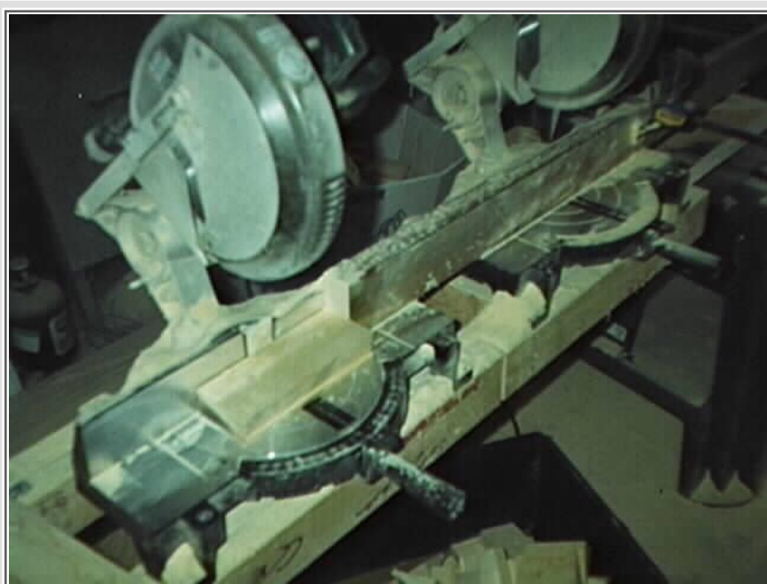
Cut predrilled wedge board in 4 inch increments
