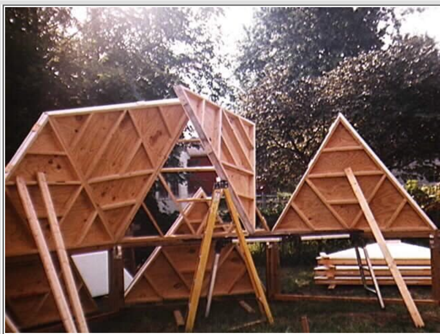
First level panels braced at 10 degree slant
