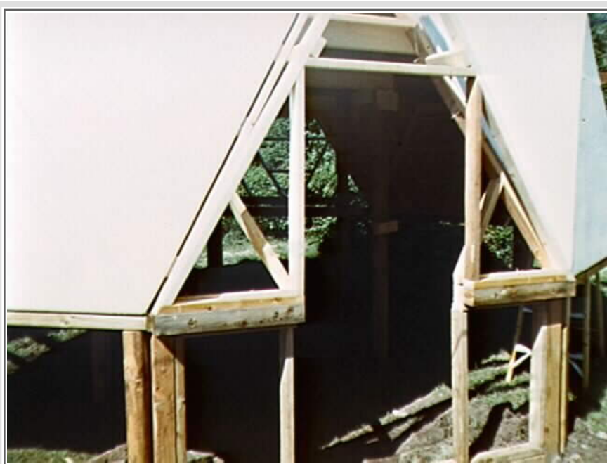
The awning support structure
