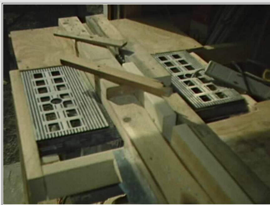
Ripping the predrilled Wedge connector boards
