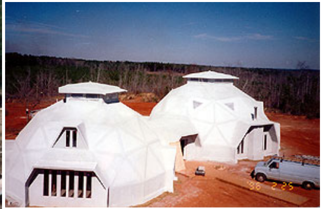
During painting using a latex house paint.
