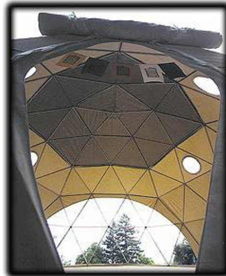
24' dome ceiling with roof and screen in place
