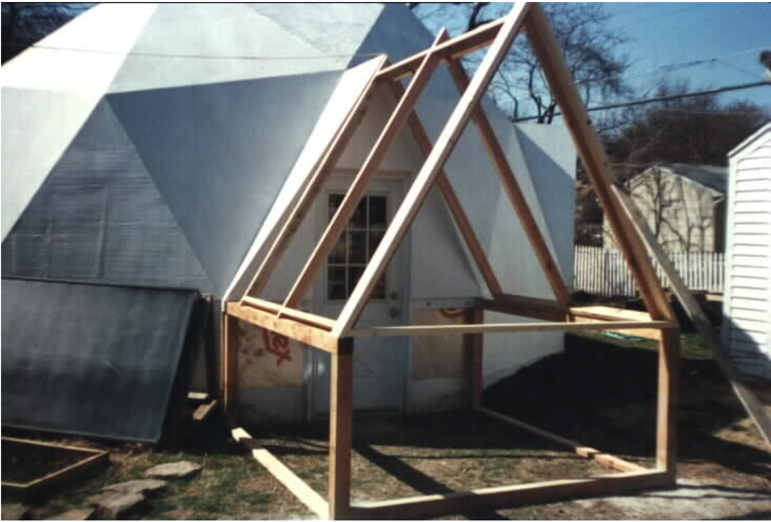
Roof Truss Installed
