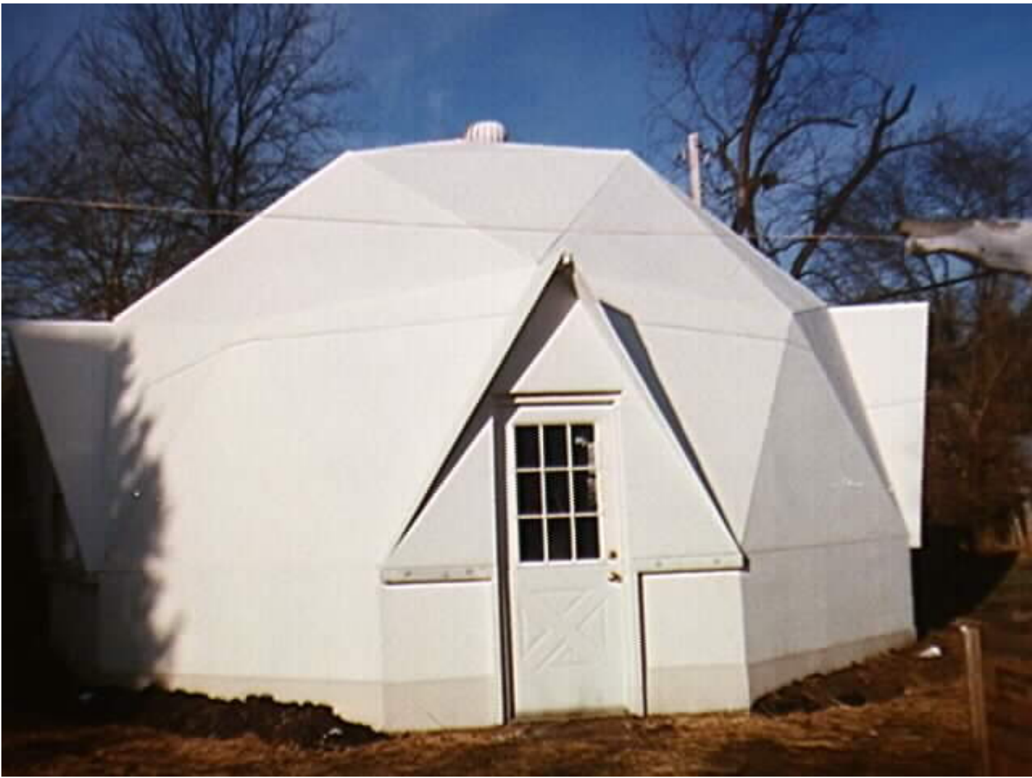
Photo of 24' Dome
