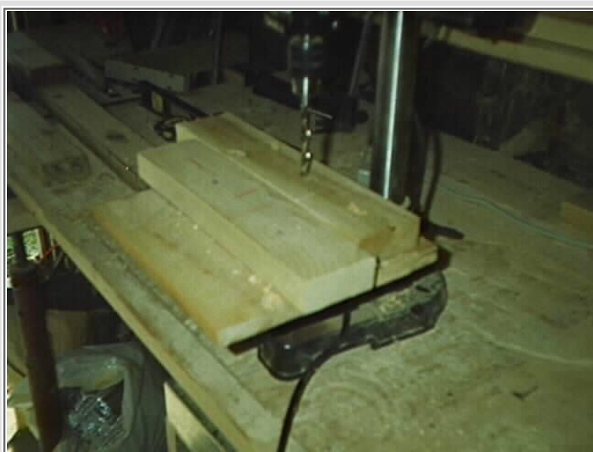
Boards being drilled to make wedge connectors
