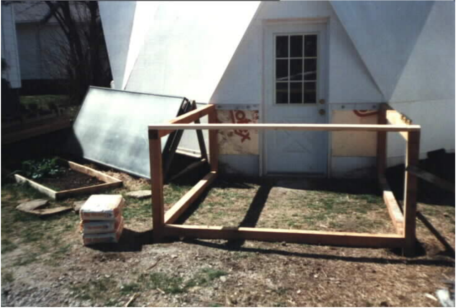
Post & Beam laid being laid out.
