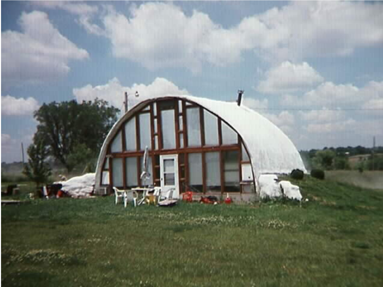
30' Diameter Lightweight Earthcontact Concrete Dome
