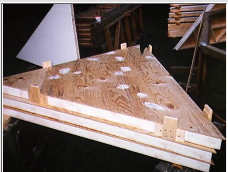
Cleats are used to position sheathing to panels
