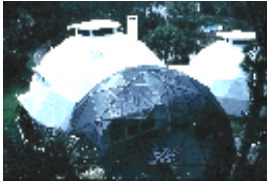
aerial view of a three dome cluster
