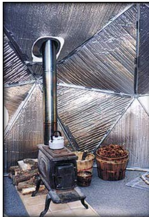
instilation of insulation
