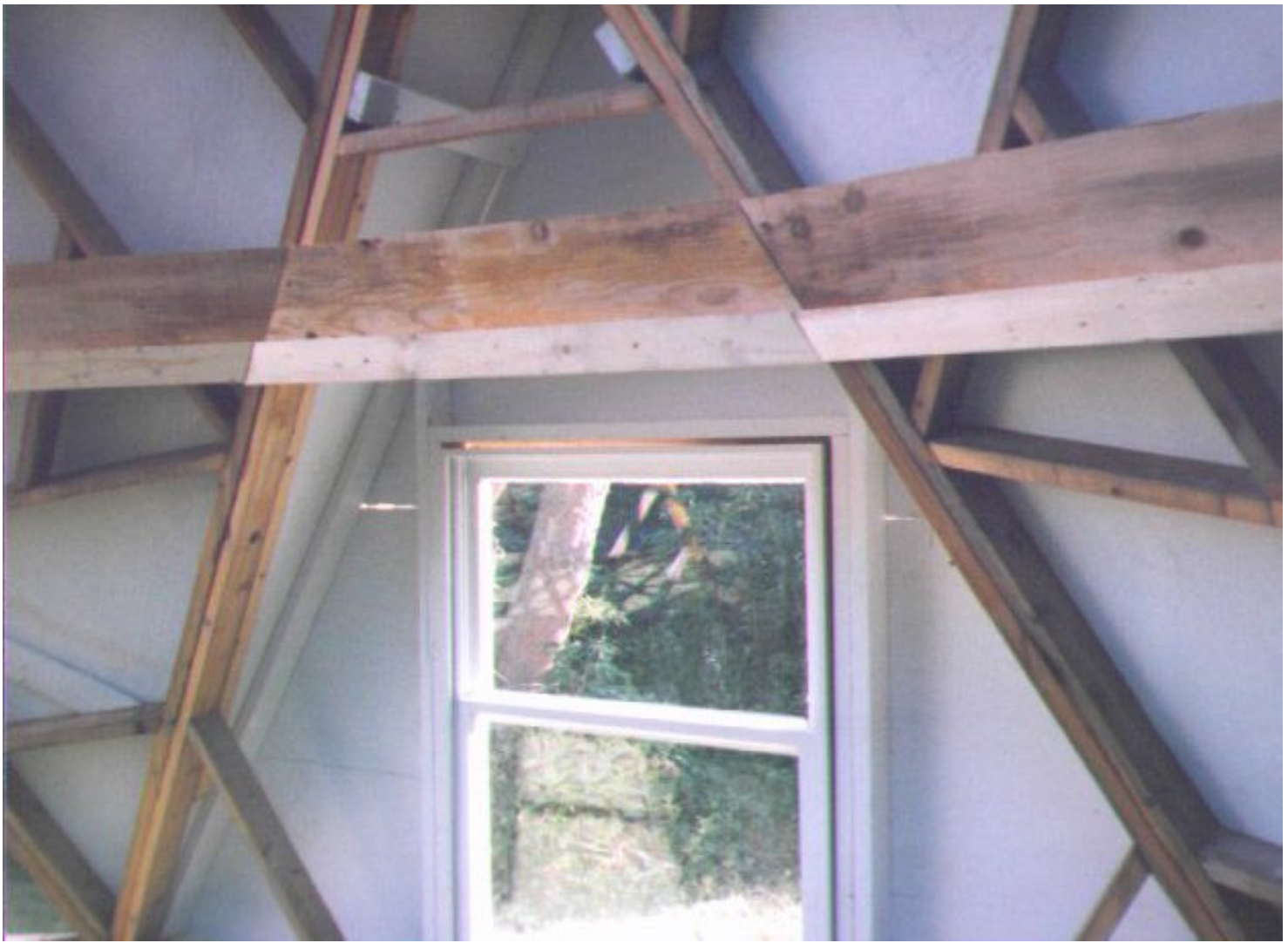
32' Dome Joist Hangers
