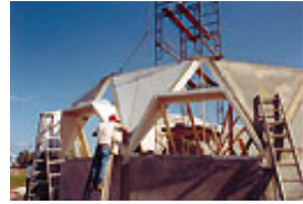
placing a panel into position
