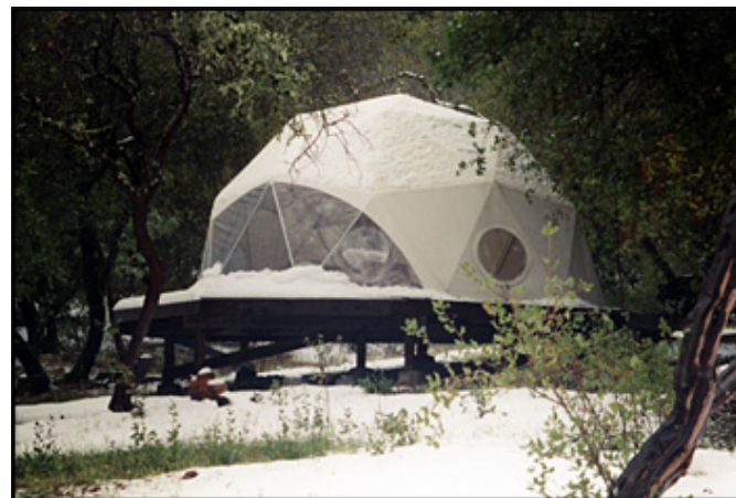
16ft with extended deck and storage underneath.
