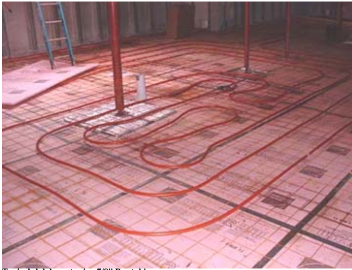
Typical slab layout using 7/8" Pex tubing
