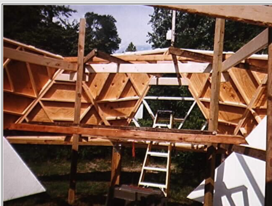
Temporary scaffold used for 2nd level panels
