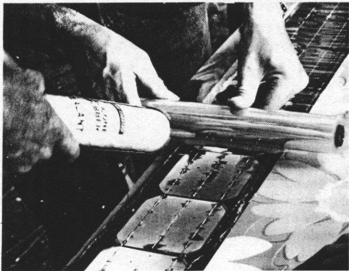
FIGURE 4.12—Coating the top of the cells with silicone and Mylar film. The Mylar film squeezes out a bead of the silicone RTV, eliminating voids and air bubbles (Courtesy Home Energy Workshop, Fort Collins, Colorado).
