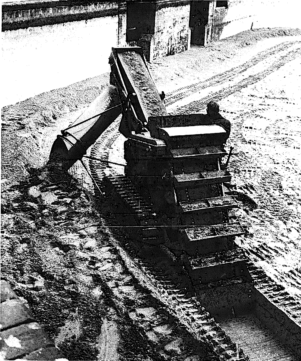
FIG. 35. TRENCHING MACHINE FOR RESANDING OPERATIONS
