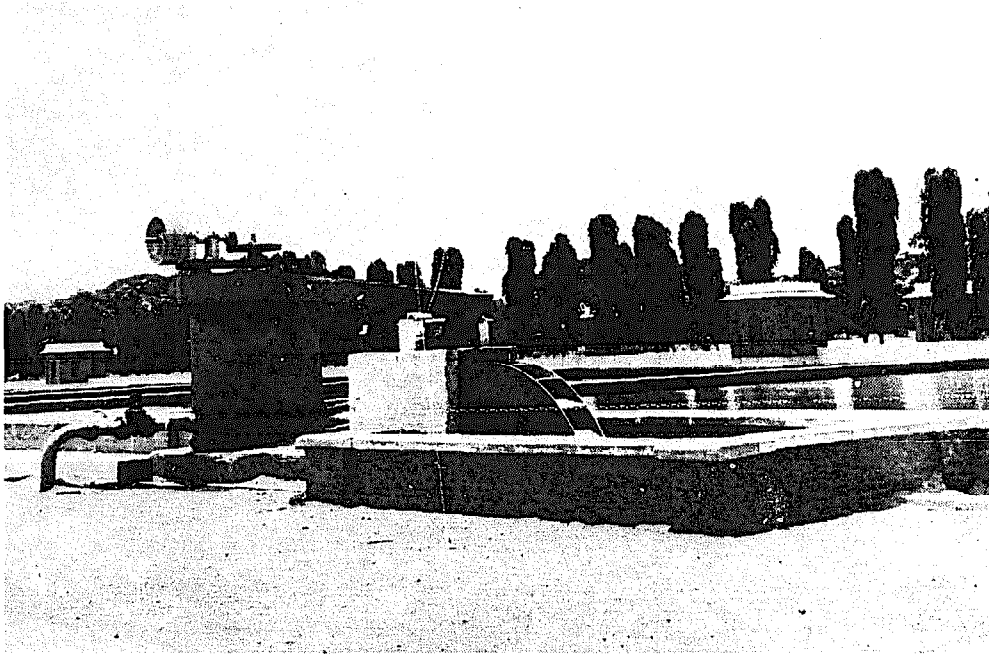
FIG. 29. GENERAL VIEW OF SAND WASHING PLANT AT MADRAS WATERWORKS, INDIA
