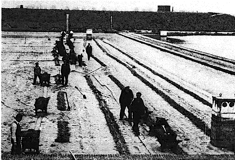
Municipal waterworks, Amsterdam
