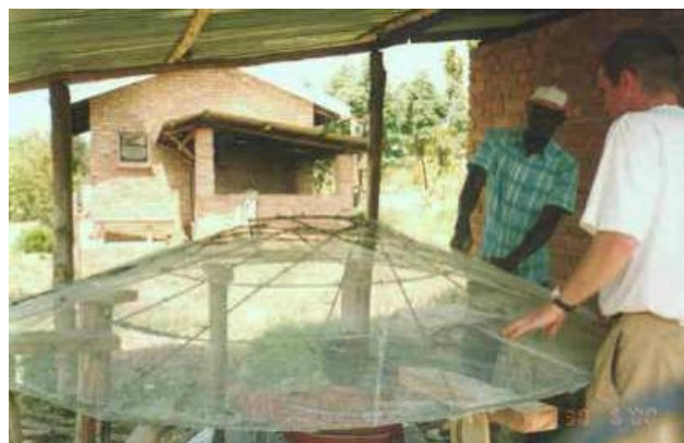
Figure 14 – the completed cover frame set on 6 supports and ready for rendering
