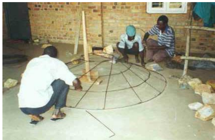
Figure 8. Assembly of the frame
