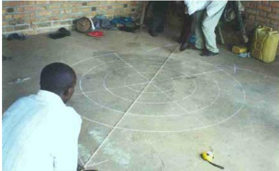
Figure 3 – Marking out the hoop diameters before bending
