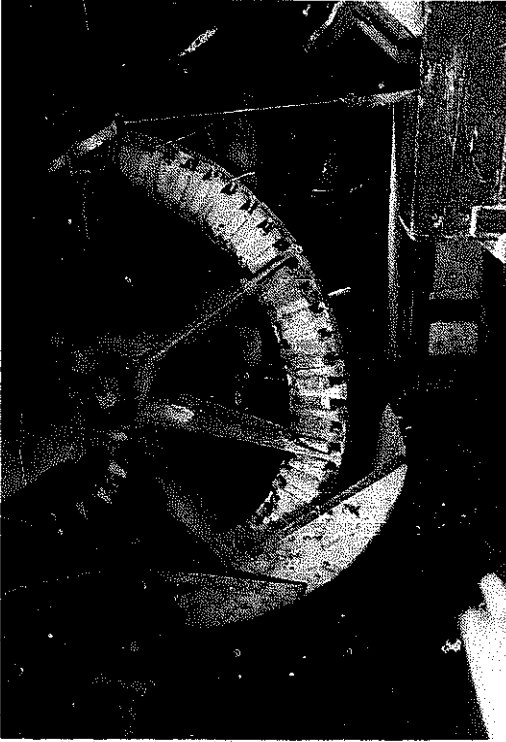
(b) Friston Post Mill, Suffolk (1938). Lever struck by tail wheel
